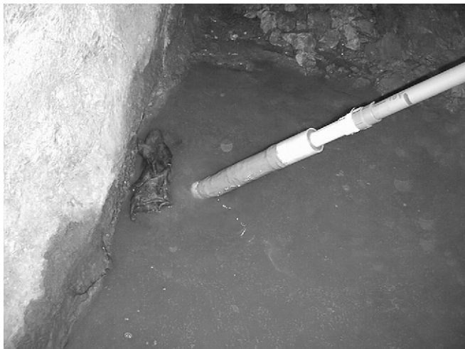
Figure 1(b): Installation of the instrument into the monitoring hole.
